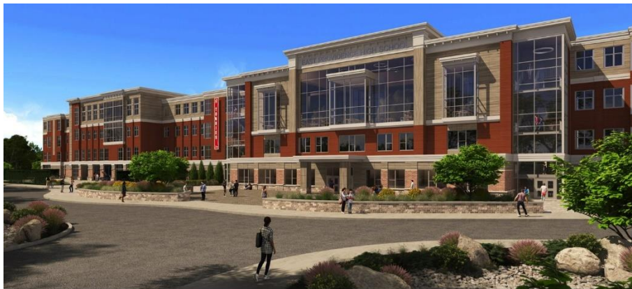
Pictured above is the fully renovated East Providence High School, which, with the help of our office, is 100% accessible.
